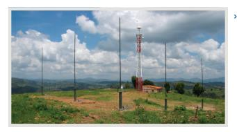
For direction finding and signal acquisition, the system is typically configured with a nine-element Model 632 monopole antenna array. Optional TCI and third-party antenna arrays also are compatible.
